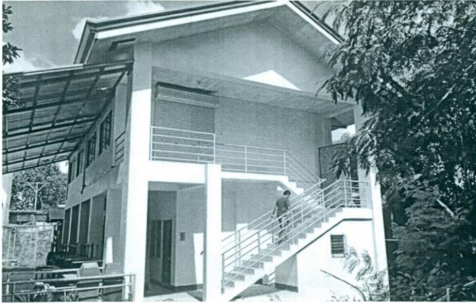
Removed and Replacement with metal Spandrel type ceiling
