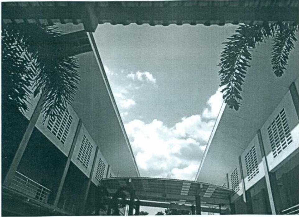
Repair of Exterior Ceiling at SRP
